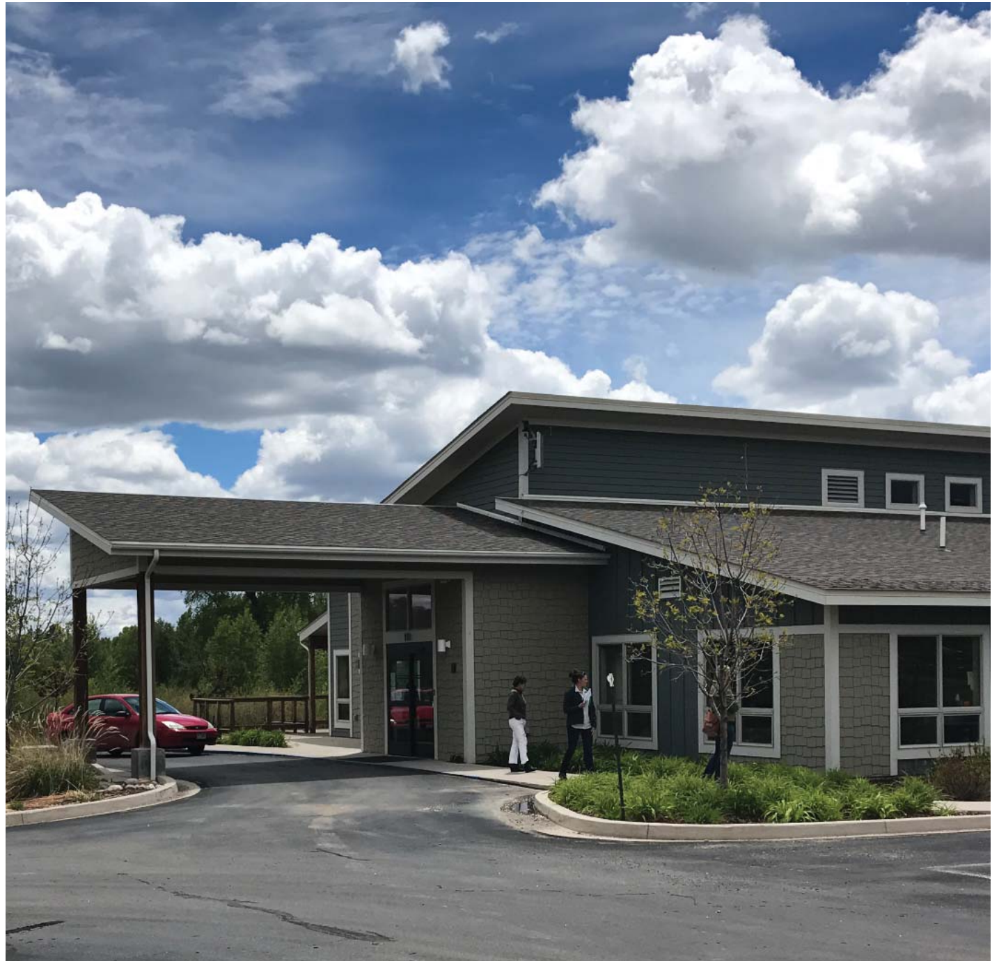
Image 45: Senior Center entrance/drop-off
