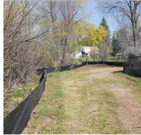
Image 35: Walking loop, with current construction silt fence
