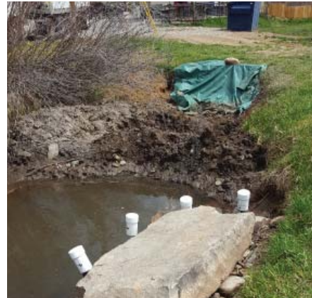
Image 70: Open irrigation collection pond at JSP
