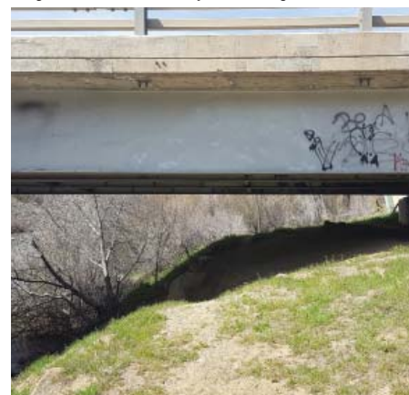
Image 69: Informal access under Hwy 160 (not maintained)
