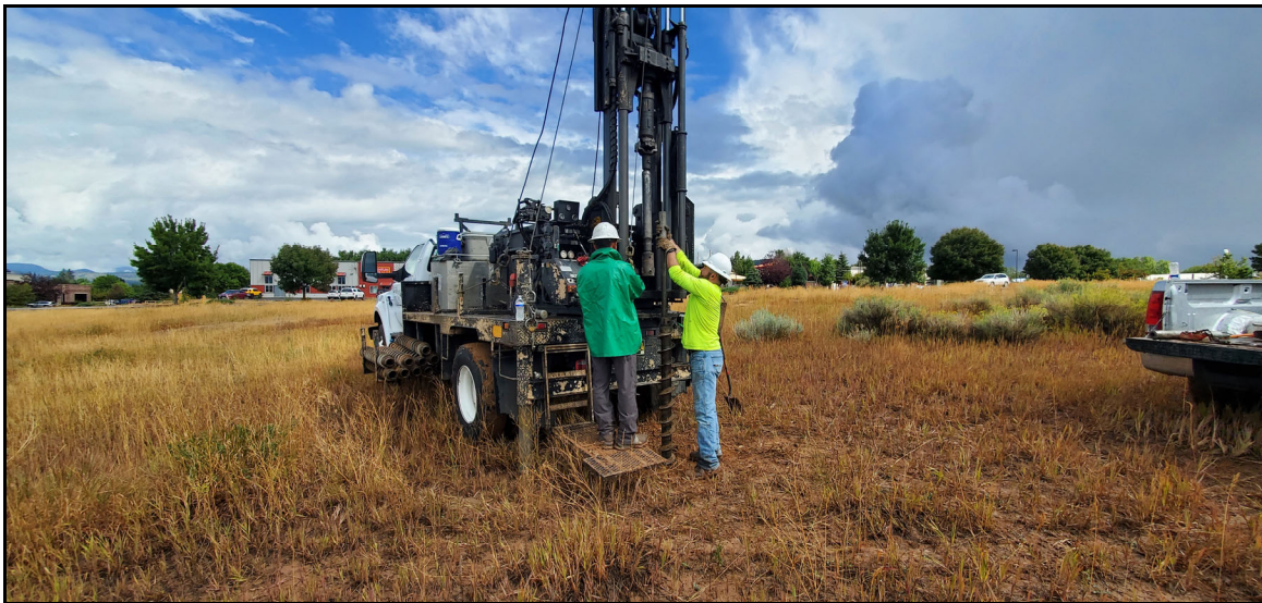
Drill Rig at Boring B-1 View Towards the Northeast
