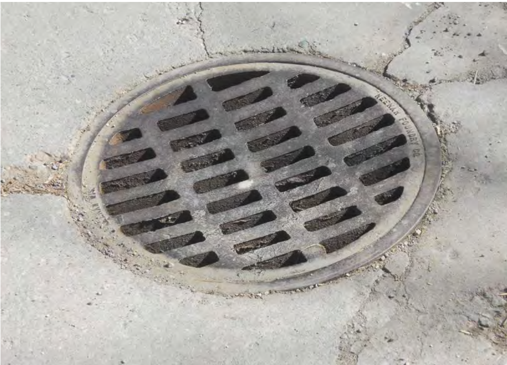
Photo 2 – Inlet – Single, 2-Ft Diameter, w/Parallel Openings
