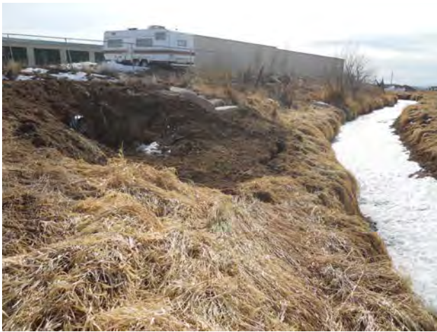
Photo 22 – Pond 24 – Outlet Pipe discharges into Irrigation Canal
