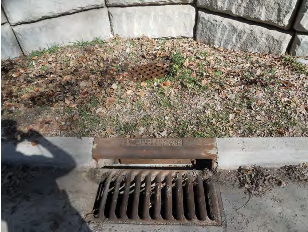
Photo 3 – Inlet – Single, 3-Ft Standard Cast iron (CI), w/Capture Vanes, and a 2-Ft Diameter, Round/Circular, w/Parallel Vanes in a sump configuration
