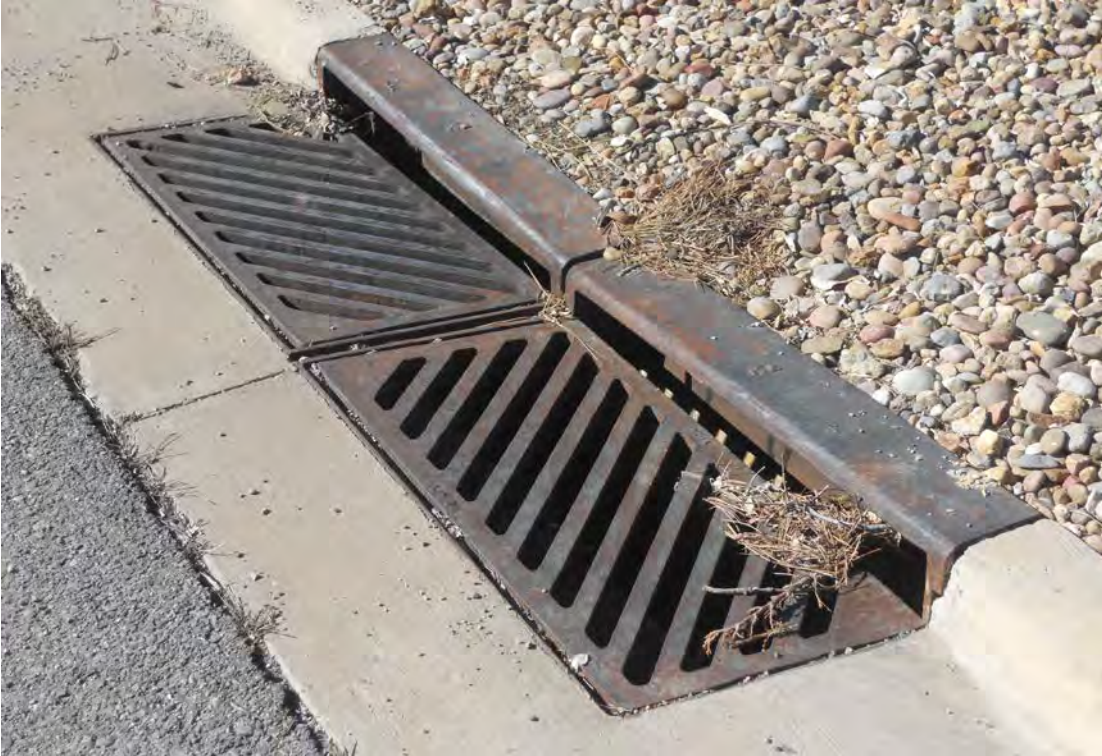
Photo 7 – Inlet – Double, 3-Ft Standard Cast iron (CI), w/Slanted/Angled Vanes
